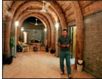
Jassim Alasida walks through the NI Adobe house on November 6. TRACEY SHELTON
