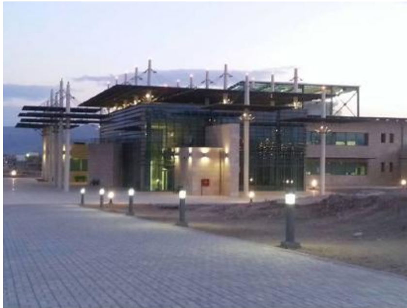
Twin Rivers Institute eco-building
