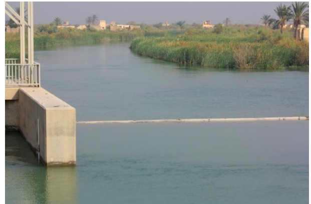
Abu-Chiwalanah Canal structure
