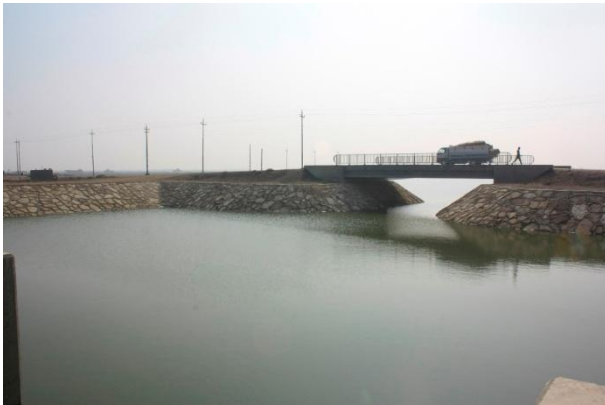
Nahar Al-Sabaa Canal structure
