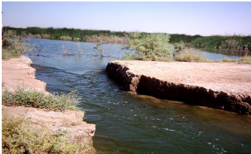
Figura 1 – Locals destroyed dyke to re-flood the Abu Zurig marsh
