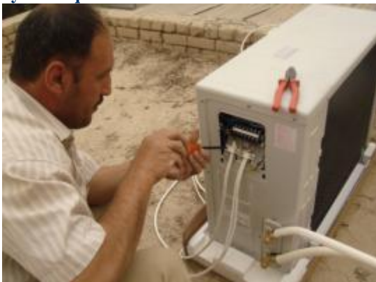
Installation of air conditioning units in Al Hammar Veterinary Center
