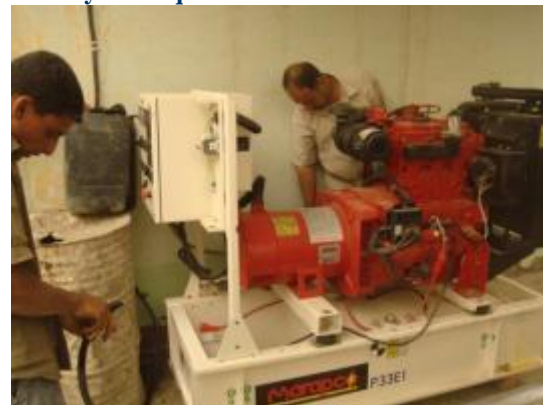
Installation of a 30 KV power generator in Al Hammar Center
