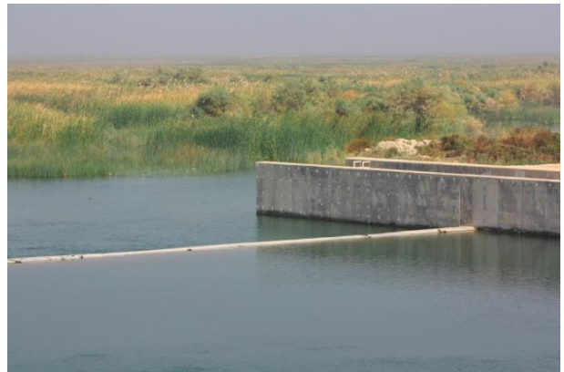
Chihalah Canal structure
