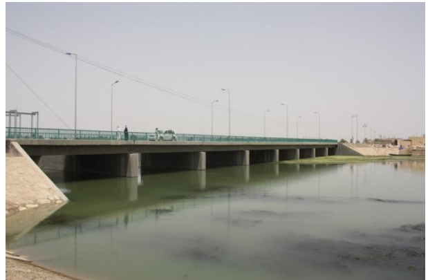
Buteira river structure
