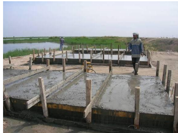
Civil works at three sites
