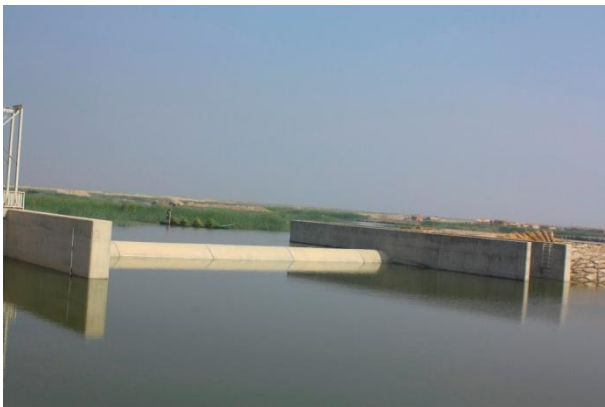
Abu-Jithaa Canal structure
