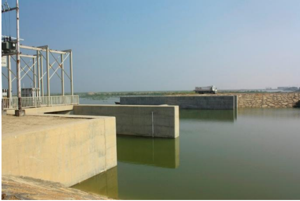
Al-Badriyah Canal structure
