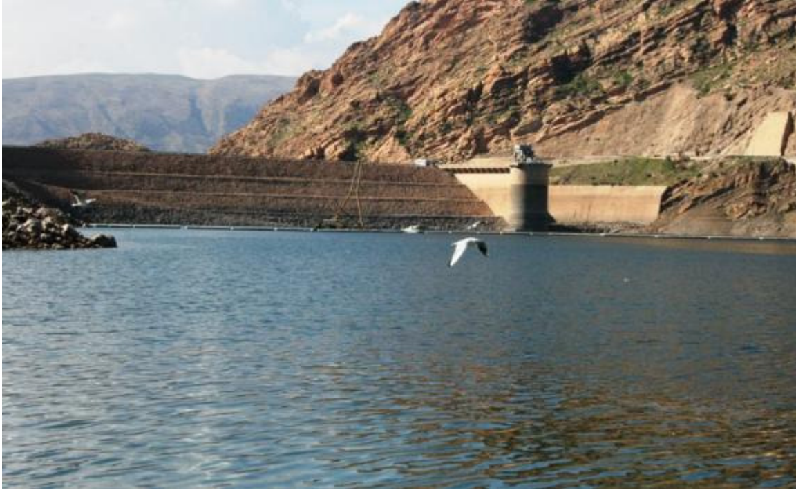
Darbandikhan Dam in winter (Photo by Hana Raza, 2010)
